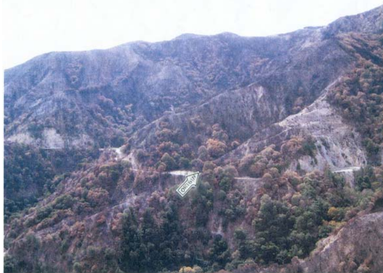
Figure 6. AERIAL VIEW OF STATION FIRE TERRAIN SURROUNDING THE ORIGIN
